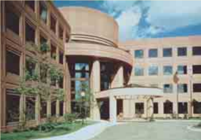
Headquarters for the Joint Commission for Accreditation of Hospital Organizations in suburban Chicago is highlighted by a stepped profile at the window recesses, as well as a heavily exposed aggregate for color and texture.
