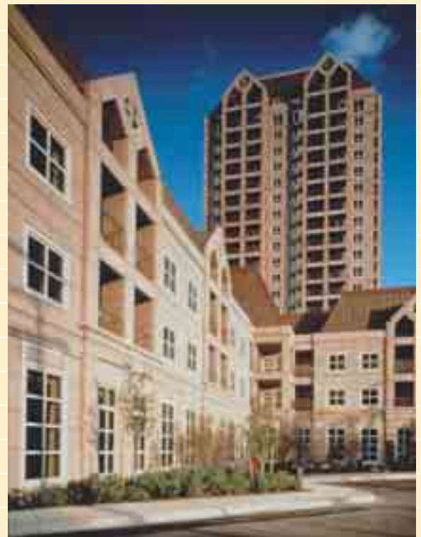
The USAA Retirement Center in San Antonio features precast concrete throughout the façade. Window panels on the low-rise structures highlight a variety of profiles and treatments, as do the balconies and window areas of the tower of the project.
