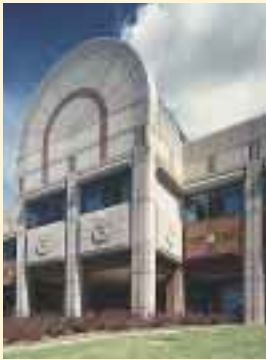
...Create a combination such as an arched roof member including a beam surround.
