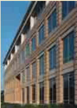
Fig. 1: The heavily rusticated panels used on 1335 Windward Concourse in Atlanta are thickened flat panels with exaggerated 3-inch quirks at the corners to create a return back into the interior of the building, giving it a perceived dimension.
