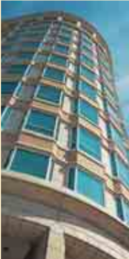
Fig. 4: This flat wall plane on the 55 Farmington building in Hartford, Conn., changes direction without corner articulation by using a shallow angle return for single casting and placing the joints at the back angles where they are de-emphasized. The shallow corner angle allows a solid cast edge.
