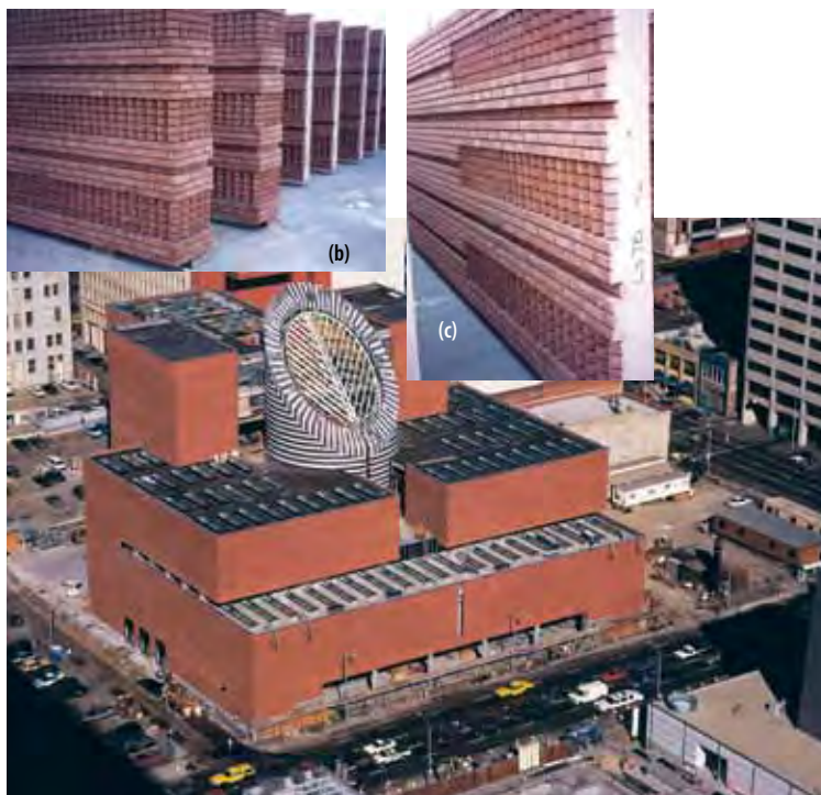
Figure 4 (a), (b) & (c) San Francisco Museum of Modern Art, San Francisco, California; Architect: Mario Botta, Design Architect: Hellmuth, Obata & Kassabaum, P.C. (HOK) Architect of Record. (Courtesy Perretti & Park Pictures)
