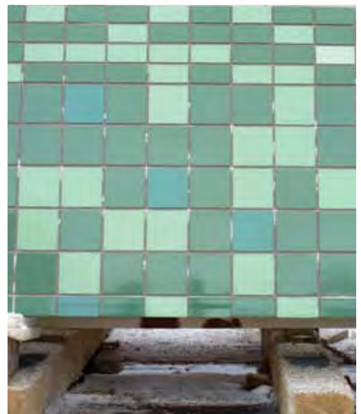
Figure 13 Mercy West Hospital, Green Township, Ohio; Architect: Ellerbe Becket (an AECOM Company), Minneapolis, Minnesota; (Photo: Randy Wilson).
