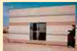
Fig. 7: Multiple mixes with acid-etched finish.
