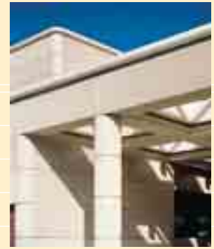
Fig. 4: Form liner and sandblasted finish.
