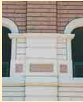
Fig. 2: Multiple mixes with retarded and sandblasted finishes.
