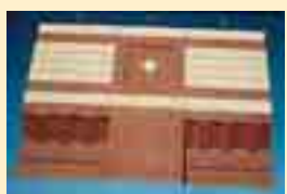
Fig. 9: Brick and acid-etched finish.
